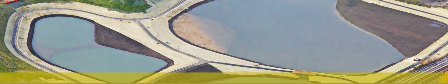
Above: Hiawatha Crossings—Stormwater Detention Ponds and Multi-Use Trail, Village of Sturtevant, WI
