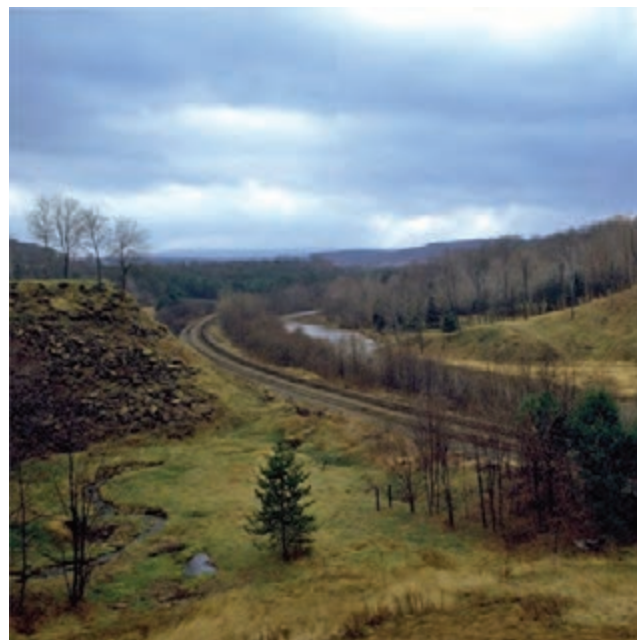
Figure 37. Current photograph of South Fork Dam depicting abutment remnants (National Park Service, 2008).
