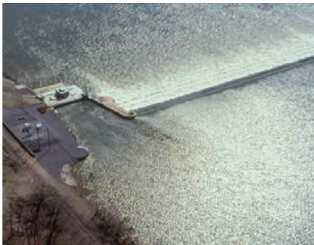
Figure 28. Aerial view of Allegheny Dam 5 and hydropower plant.
