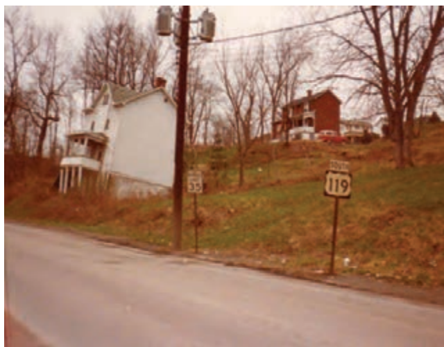
Figure 42. House damaged by sinkhole subsidence, Connellsville, PA (photo by R. Turka, 1979).
