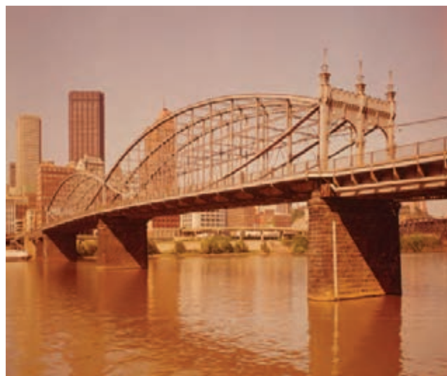
Figure 49. Smithfield Street Bridge in downtown Pittsburgh: Historic American Engineering Record collection (Cridlebaugh, 1999).
