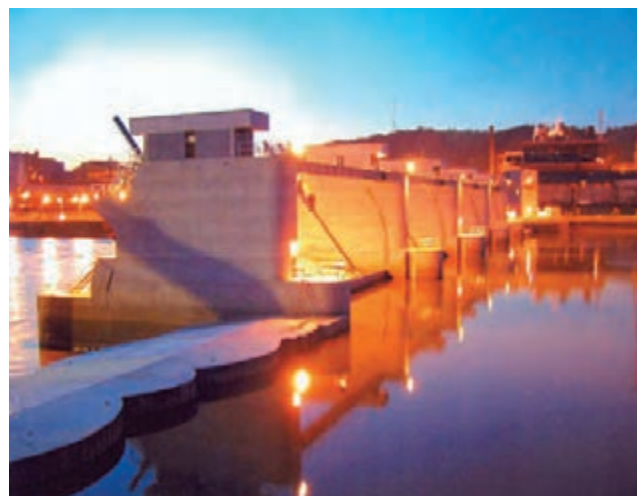
Figure 60. Completed Braddock Dam in 2004 (courtesy of the U.S. Army Corps of Engineers, Pittsburgh District).
