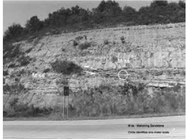
Figure 30. Typical low-angle thrust fault near Pittsburgh (photo courtesy John Harper, Pennsylvania Geological Survey).
