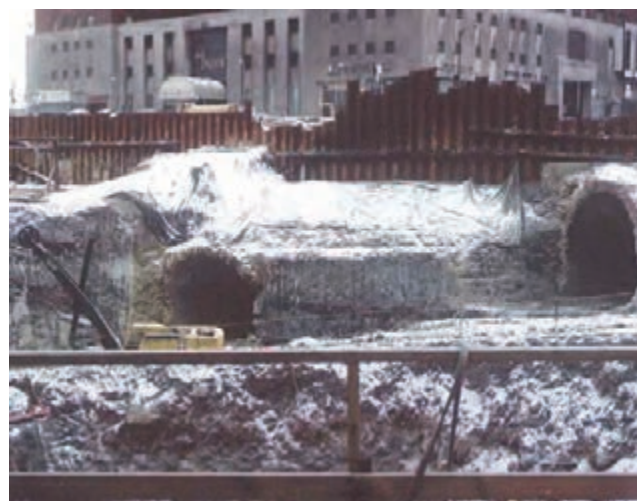
Figure 44. Tunnels exposed during USX Tower construction (Rathke, 1968).
