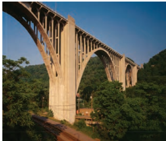
Figure 51. George Westinghouse Bridge: Historic American Engineering Record collection (Cridlebaugh, 1999).
