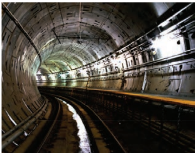
Figure 56. Interior of the completed North Shore Connector Tunnel (photo courtesy of Port Authority of Allegheny County, 2012).
